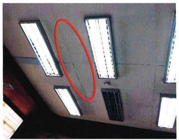
Existing ceiling boards and wooden frames infested by termites. Wooden frames are damaged and may have tendency to collapse if not replaced.
