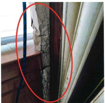
Dilapidated accordion wall, headers and side walls. Need to be replaced immediately.
